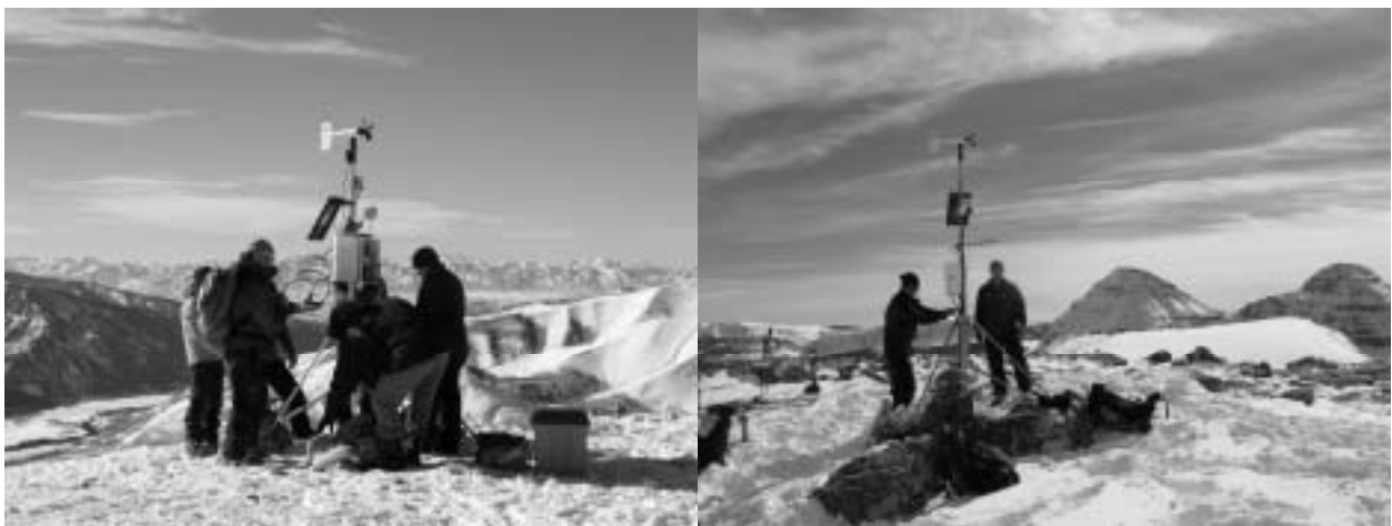
National Weather Service personnel Greg Wallace and Al Martinelli along with the Park City Powder Cats guides help install weather instrumentation on Windy Peak. Once this site was solid and running flawlessly, Ted Scroggin, Justin Cagle and Craig Gordon installed another site on Lofty Peak near the Mirror Lake Highway. An automated snow site by Mirror Lake will be added this winter.
